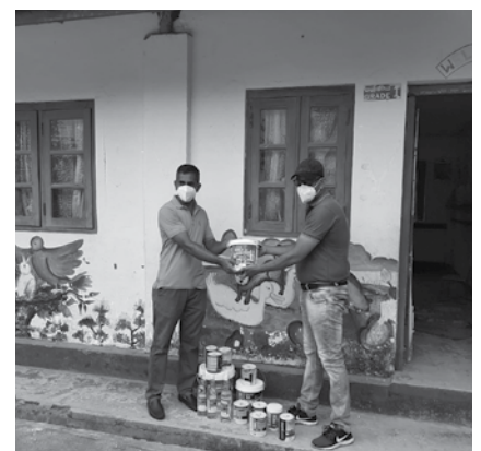
Buildings of Morothotayawatte School, located in Hatton, were painted by Broadlands Tea Factory
