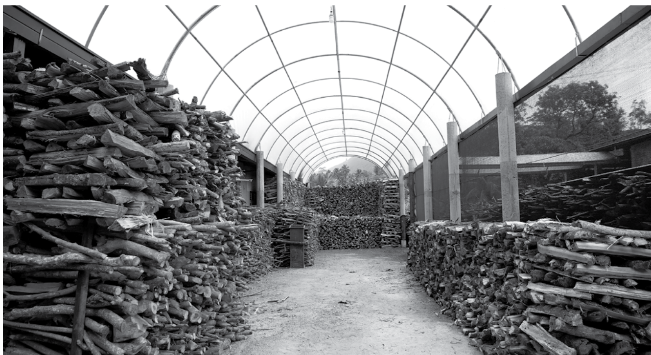
Fast drying firewood shed at Neluwa Tea Factory
