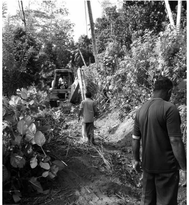
Clearing a village access road at Kurupanawa
